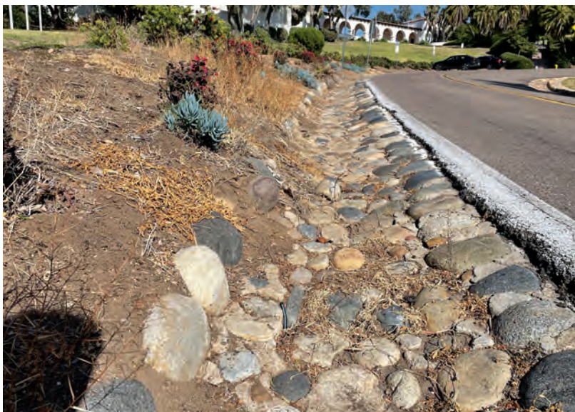
Presidio Park historic cobblestone curb and swale. Photo by Barry E. Hager.
